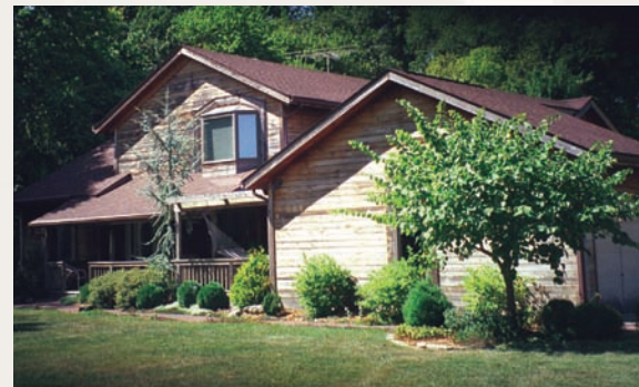
Before: Cedar-sided home in Highland, IL, before Dryvit EIFS renovation.
