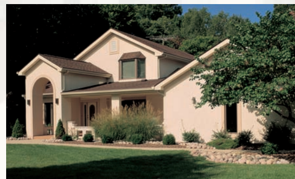
After: Using the same building footprint, the Dryvit EIFS cladding achieves a 22% energy savings (see chart above).
